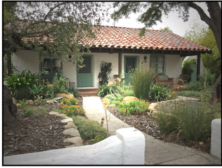
The Aliso Street Adobe is a Mills Act property.
